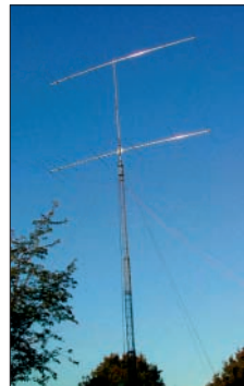
● Two Trident 7-element long boom 50MHz Yagis spaced 6.7m (22ft) apart - 23m (75ft) high at the Mike G3SED's QTH.
