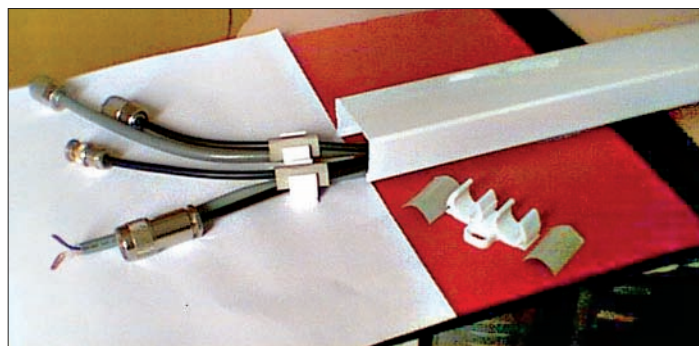
● Fig. 2: A suitable replacement for surface mount electrical trunking may be found in a plumbing centre (See text for more detail).
